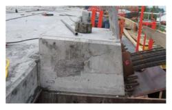
Fig. 3. Damaged cantilever no. 4 after prestresing
