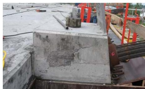
Fig. 3. Damaged cantilever no. 4 after prestressing
