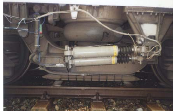
Figure 4: View of the dampers on the I.C.E. II train with attached sensors and cables
