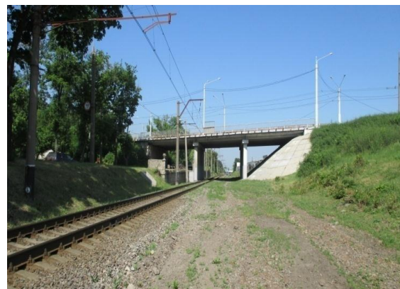
Fig. 2. Over-bridge main view
