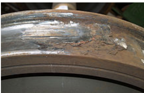
Fig. 1. Wheel-flat on a wheel surface
