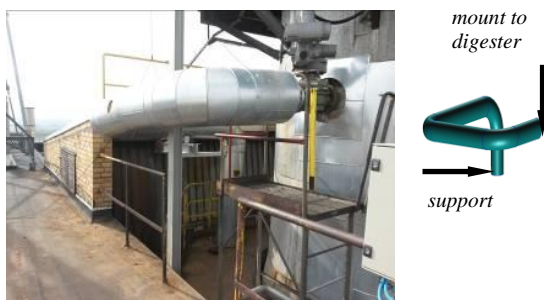
Fig.10. The upper pipe section mounted to the digester
