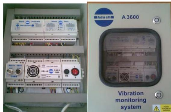
Fig. 2. Vibration monitoring system ADASH 3600
