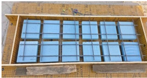
Fig. 7. Top view showing the reinforcement meshes and polystyrene blocks.
