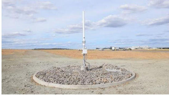
Fig. 2. GBAS reference station [8]
