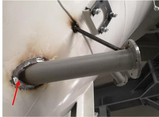
Fig. 8. Weld repair and support installation
